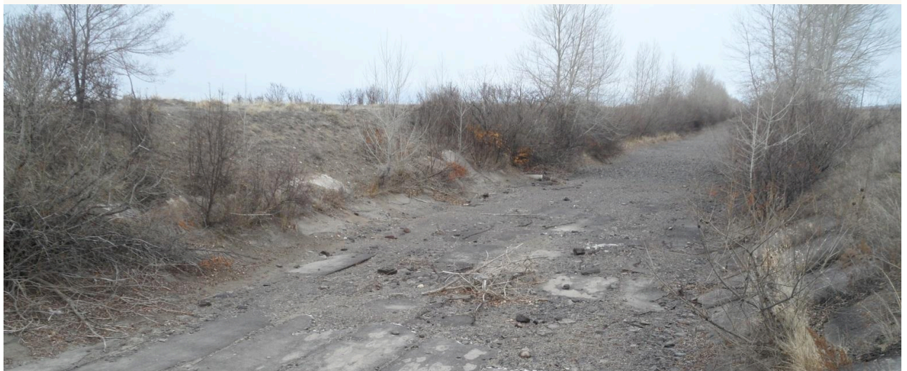
Photograph 21. The Koibal Main Canal in autumn, after seasonal drainage.
