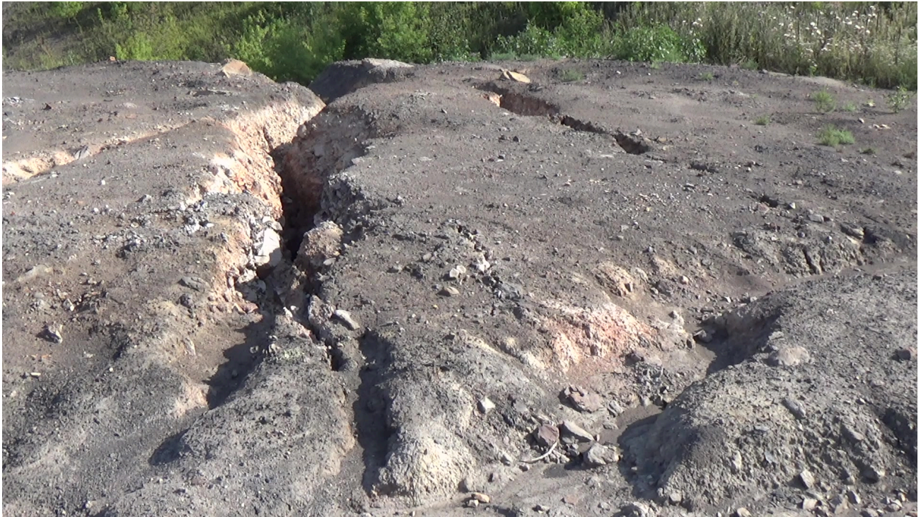
V04. A large fissure in exposed ground. Kiselevskaya mine field, 13 August 2019. Frame from Natalia Zubkova's video C0040.MP4 , timecode 00:00:16. Natalia attributed the location; the file contains no GPS data. The frame shows the condition of the surface but does not establish what caused the fissure.
