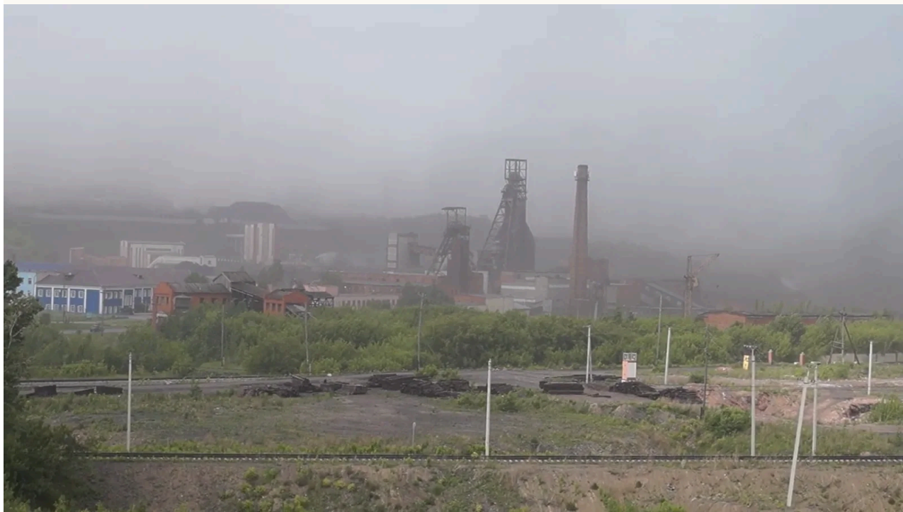
Industrial facility in haze. Kiselevsk, 2020. Photo: Smogman.
